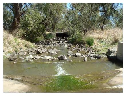
Picture 3-6 Typical rock-ramp fishway structure
