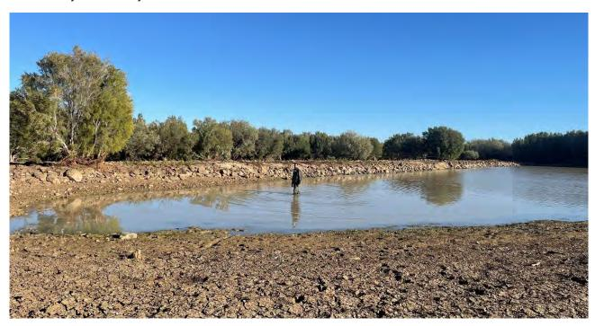
Picture 5-1 Insufficient water depth for boat-launch upstream of Fairmont Weir (TRPE7)
